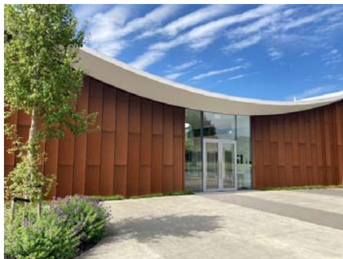
View from Villa Maria College driveway
